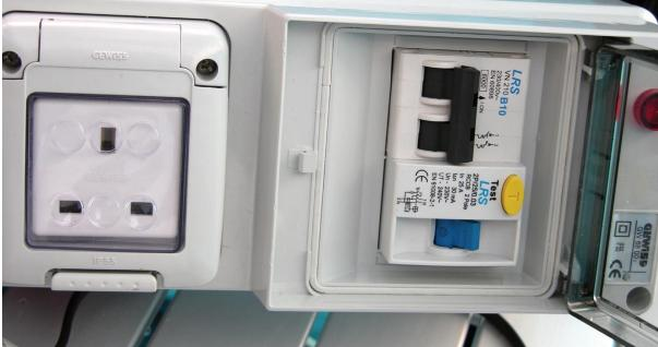
Use only proprietary hook-up equipment with RCD's and circuit breakers and test them regularly
