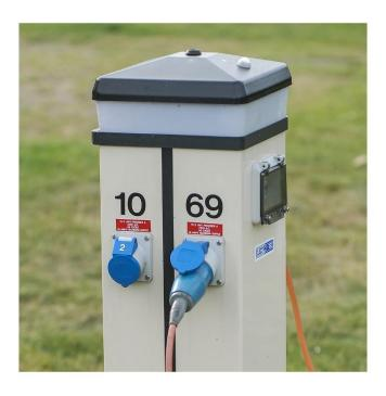
A typical electrical hook-up bollard Minimise the risks
